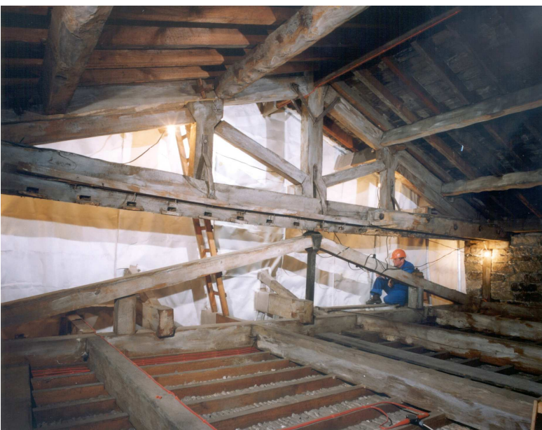
TBA Firefly Plus 60 Cavity Fire Barrier fitted within the historic Chatsworth House indicating the versatility of the system – suited to both old and new structures.
