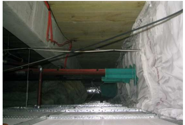
TBA Firefly Plus 60 Cavity Fire Barrier installation provide Permanent Passive Protection
