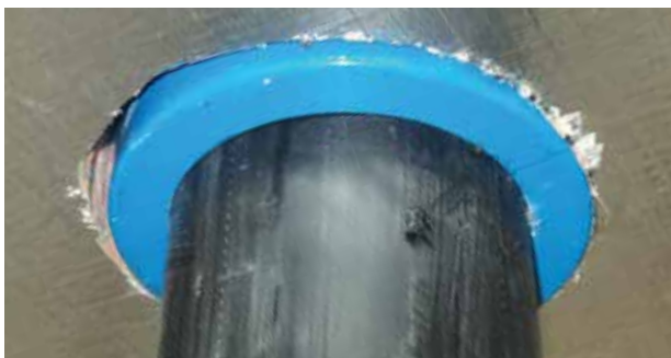
Figure 7 Penetration example - Kingspan Kooltherm ® K10 G2 Soffit Board installed tight around the fire collar and HDPE service pipe.
