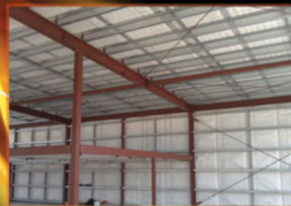
SES Building 2012 NSW
