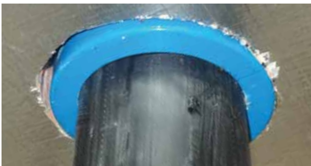
Figure 7 Penetration example - Kingspan Kooltherm® K10 FM G2 Soffit Board installed tight around the fire collar and HDPE service pipe.
